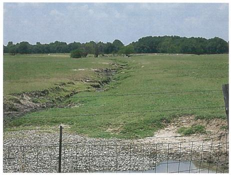
Photograph 7.4 Cleared and degraded riparian corridors along streams at the proposed mitigation site
