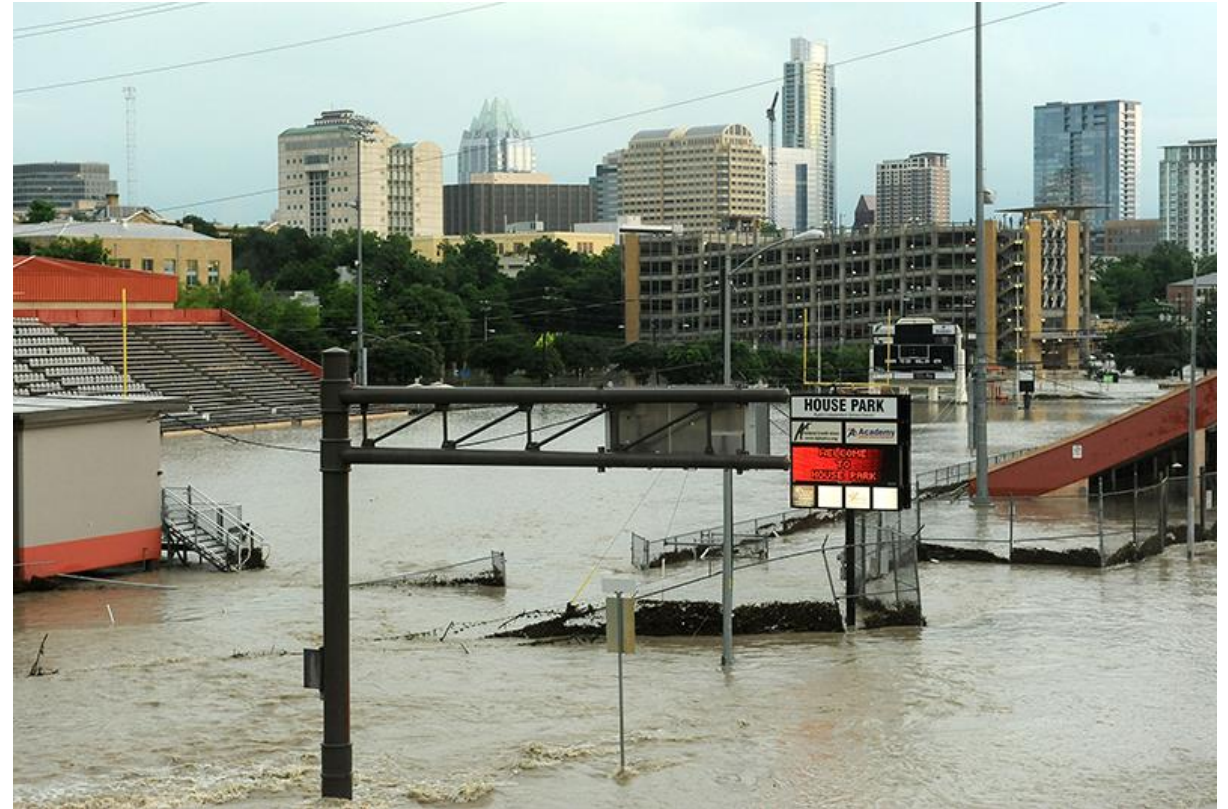
Shoal Creek flooding, Austin, TX. Image: TWDB
