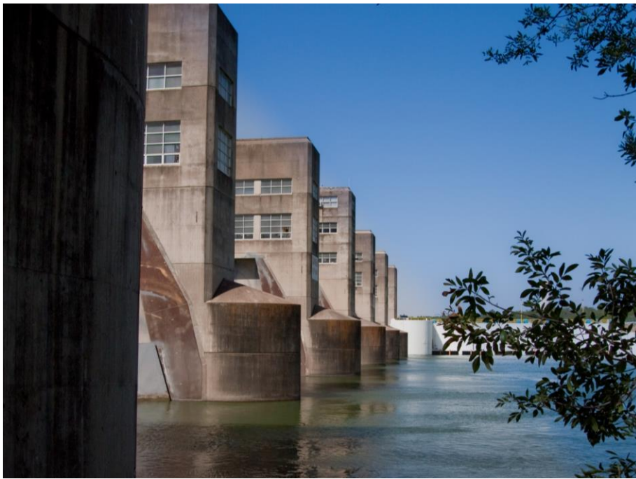
Anzelduas Dam on the Rio Grande near Mission, TX. Image: TWDB
