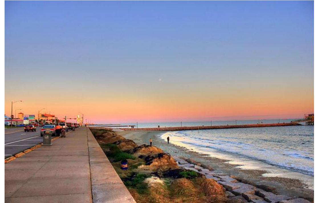
Galveston Seawall, a structural flood mitigation solution. Image by Yinan Chen CC-PD
