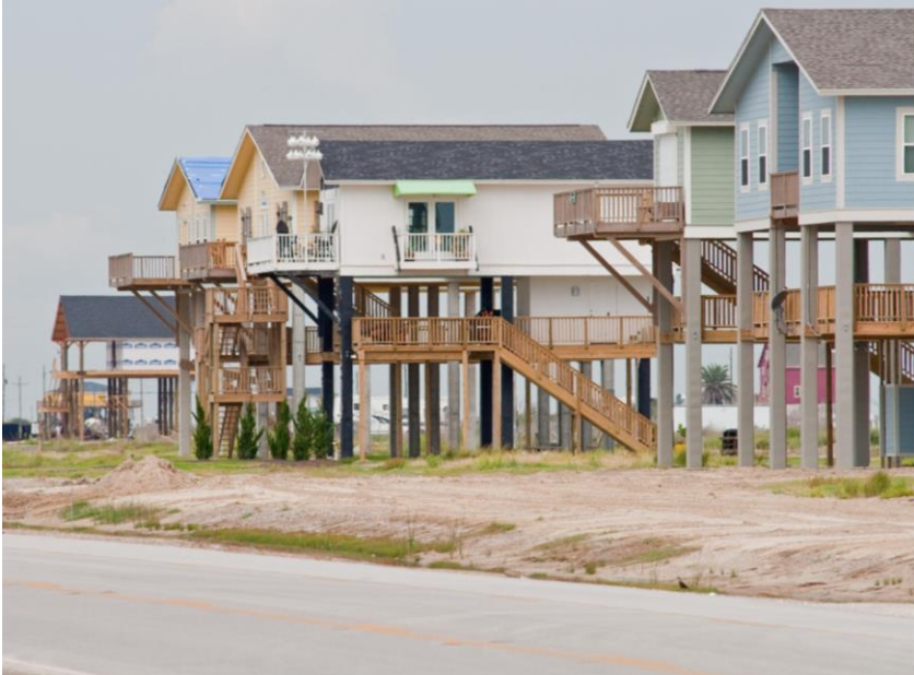
Homes that survived the ~20-foot-high storm surge of Hurricane Ike in Bolivar Peninsula, near the community of Caplen.
