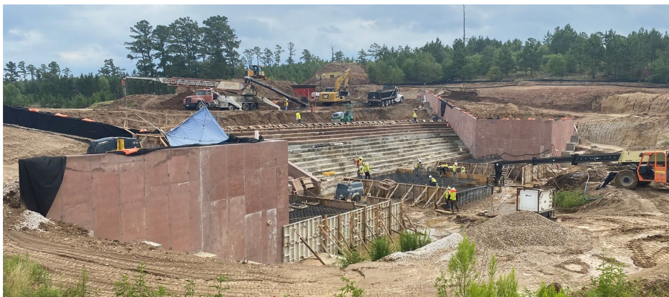
Reconstruction of the Bastrop State Park Dam
