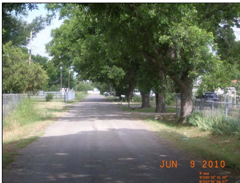
Photo 1 - Looking west at the bar ditches along Duty Lane.
