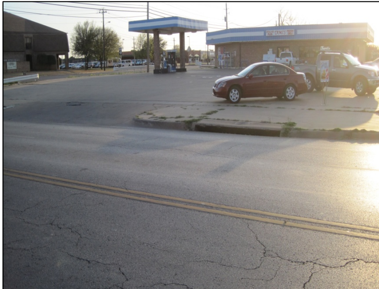
Photo 2 - Existing inlet on Rhea Road
