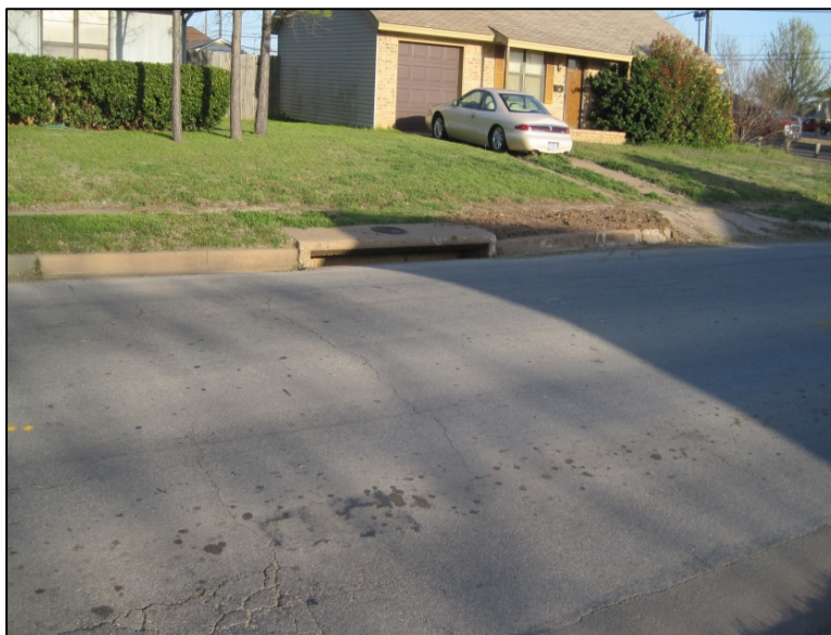
Photo 1 - Existing inlet located on Rhea Road
