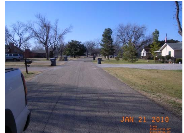
Homes at street level with no road drainage.
