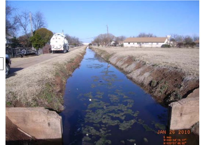
Looking northwest along the irrigation canal east of Sierra Madre Dr.
