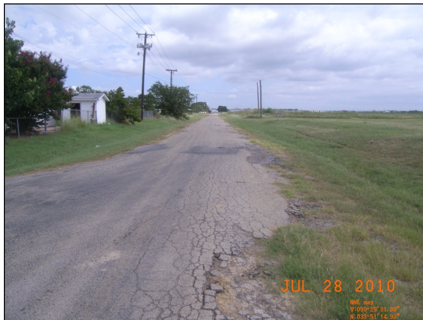
Photo 1 - Looking south at bar ditches on Ditto Lane.
