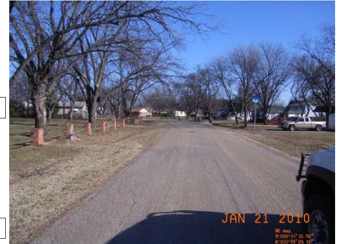
Wichita Gardens typical street section with no curb and gutter and very shallow road side swales.
