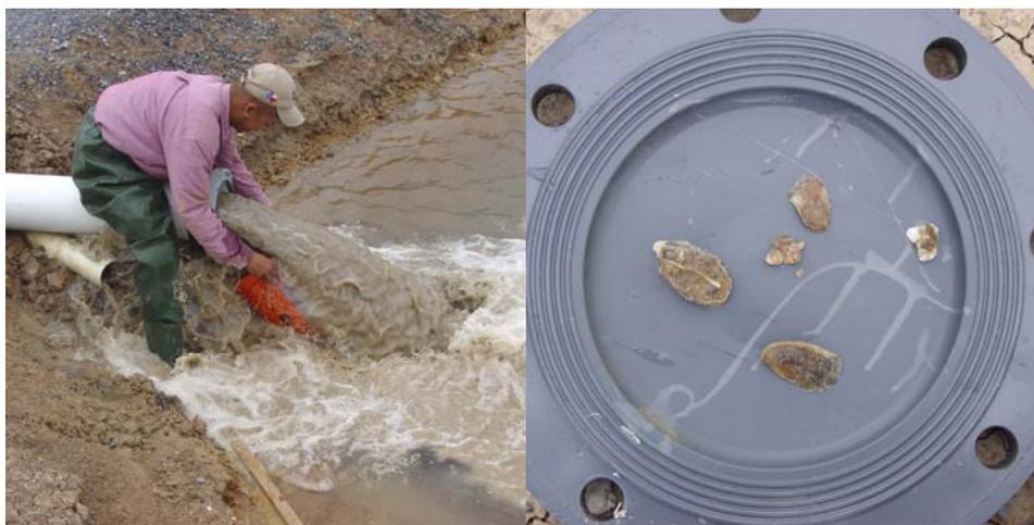
**Figure 4-2: Photograph of sampling for shell fragments and other large debris being discharged during flushing of the raw water manifold (left) and examples of some shell materials recovered (right).**
