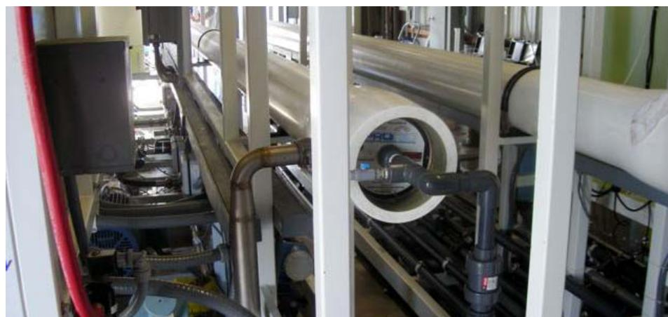
**Figure 3-45: Photograph of seawater RO pressure vessels used during the Pilot Study.**
