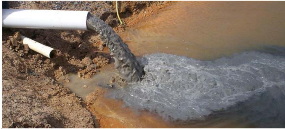
**Figure 4-1: Photograph of discharge into the lagoon from flushing the raw water manifold. Flushing was periodically required to eliminate the buildup of sediment and other debris in the manifold line.**
