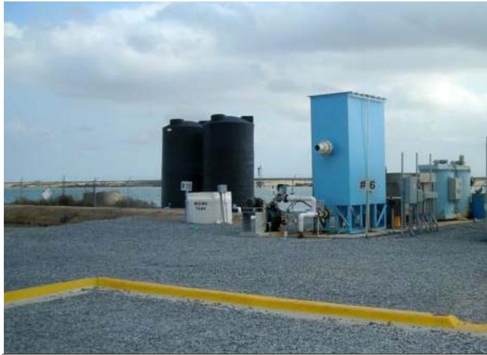
**Figure 2-6: Photograph of the Eimco conventional pretreatment system.**
