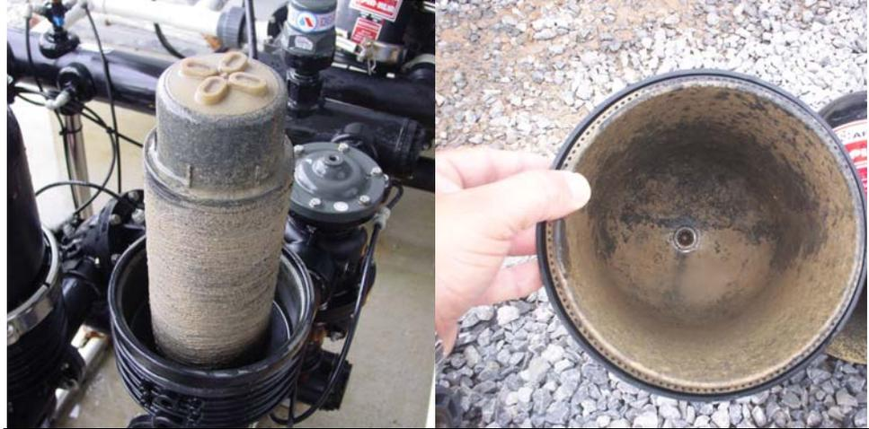
**Figure 3-13: Photograph of sediment buildup in the discs (left) and hood (right) of one of the GE Zenon Arkal units.**
