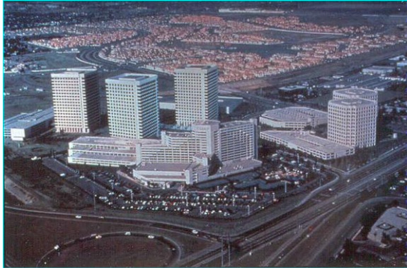
Figure 20. Dual-plumbed office building (Source: Irvine Ranch Water District)
