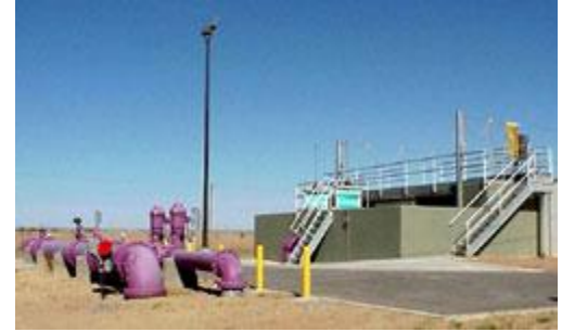
Figure 8. Roberto R. Bustamante Plant (Source: El Paso Water Utilities)
