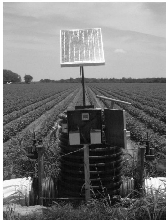
Surge valve with solar-powered controller.
