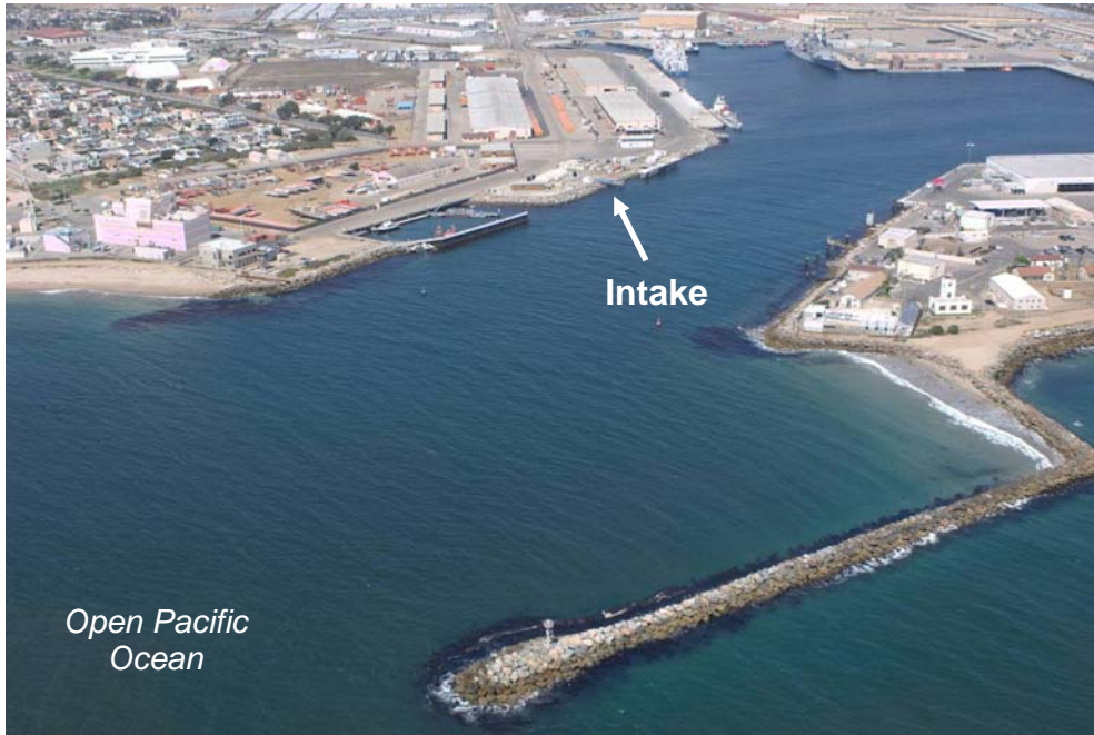
Figure 3.1 Raw water intake at Port Hueneme
