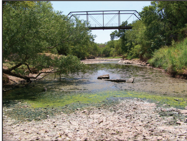
August 6, 2011, 0 cfs – downstream
