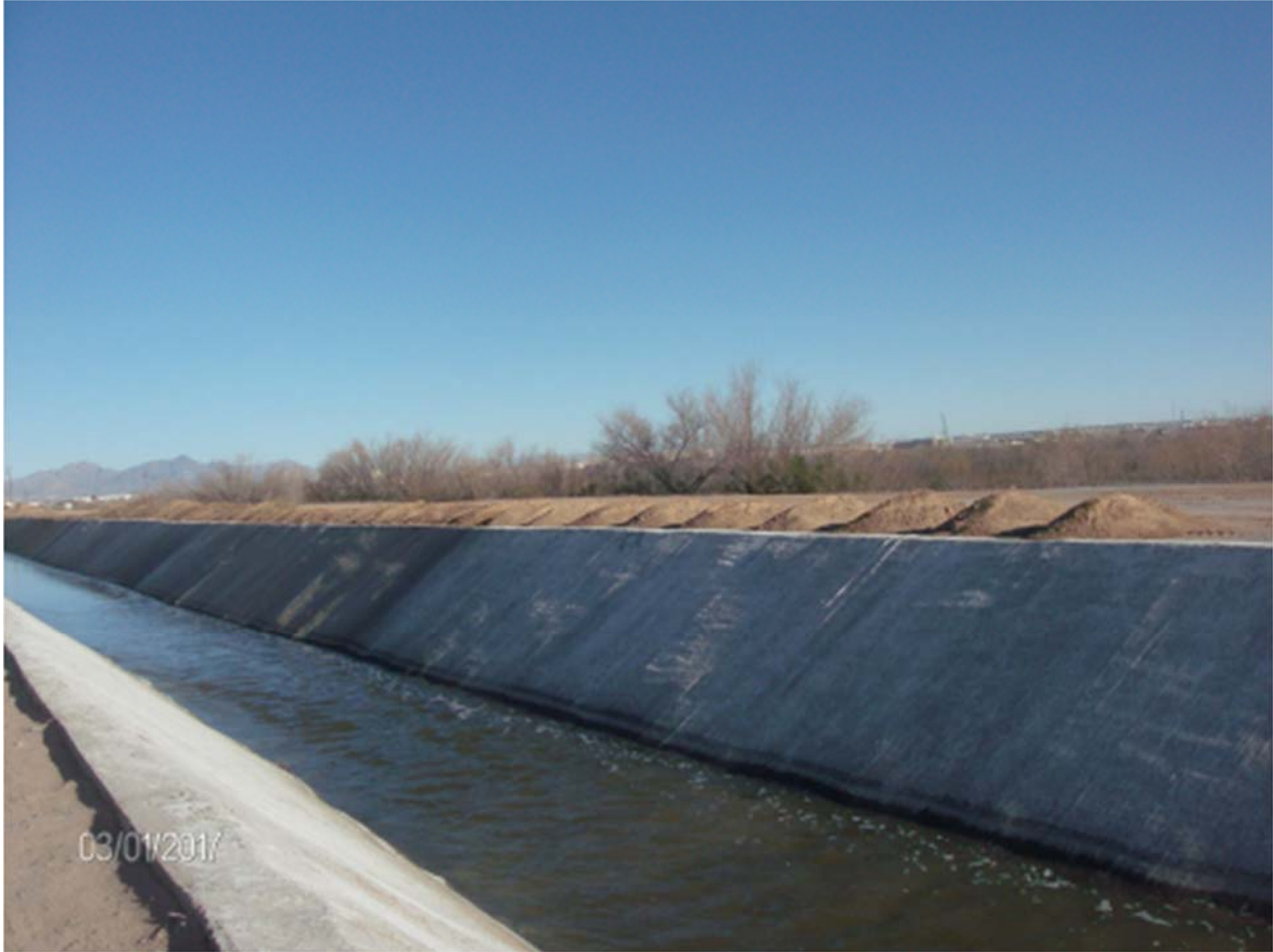
Completed concrete lining downstream from wastewater discharge structure. Photo dated 3/1/2017.
