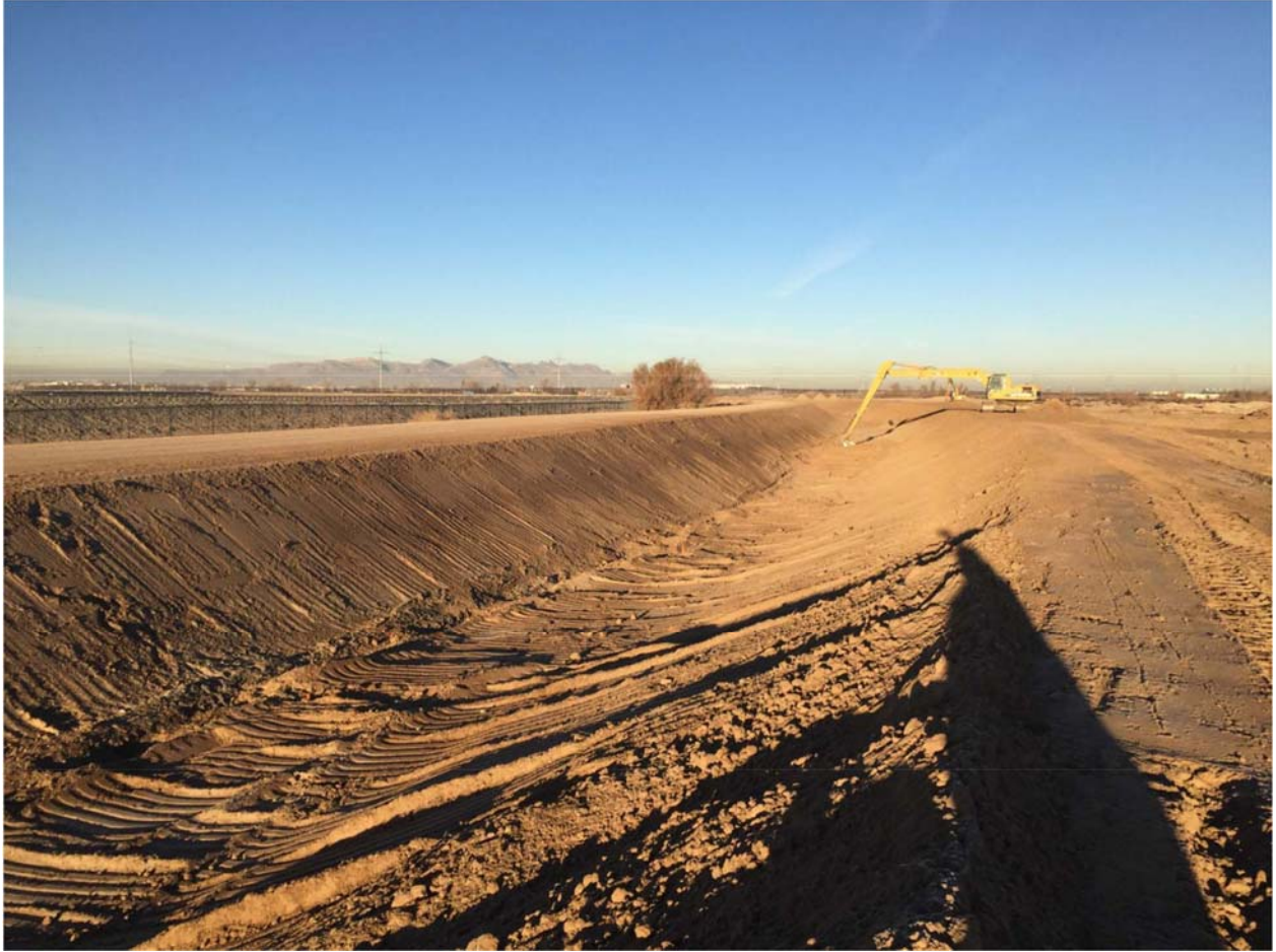
Location 5. Continued earthwork and canal shaping. Photo dated 1/21/16.
