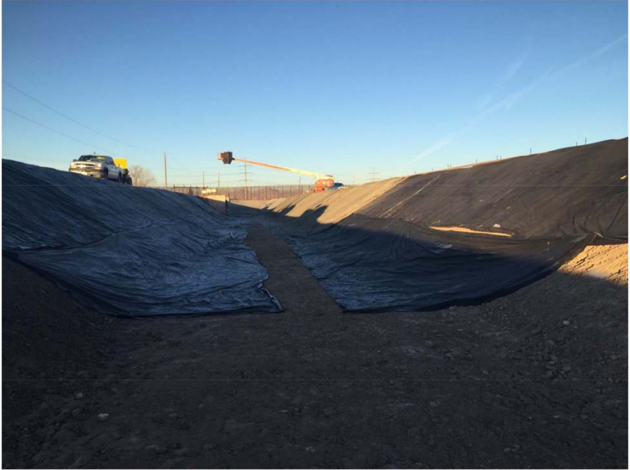
Location 3. Geofabric liner placed on canal sides. Photo dated 1/21/16.
