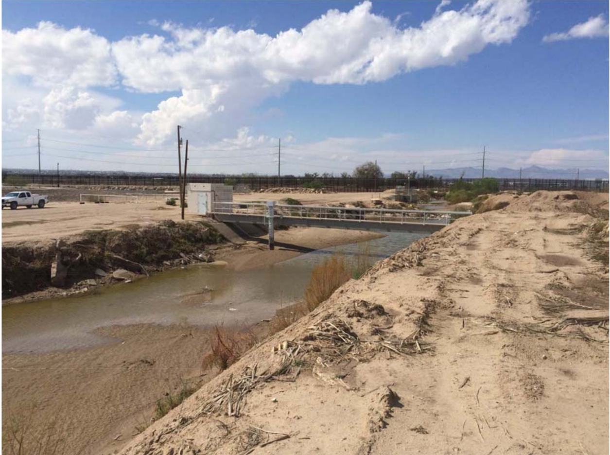
Location 4. Pre-construction photo dated 10/21/15 of the Riverside Canal heading metering bridge. The canal was dried before construction began.
