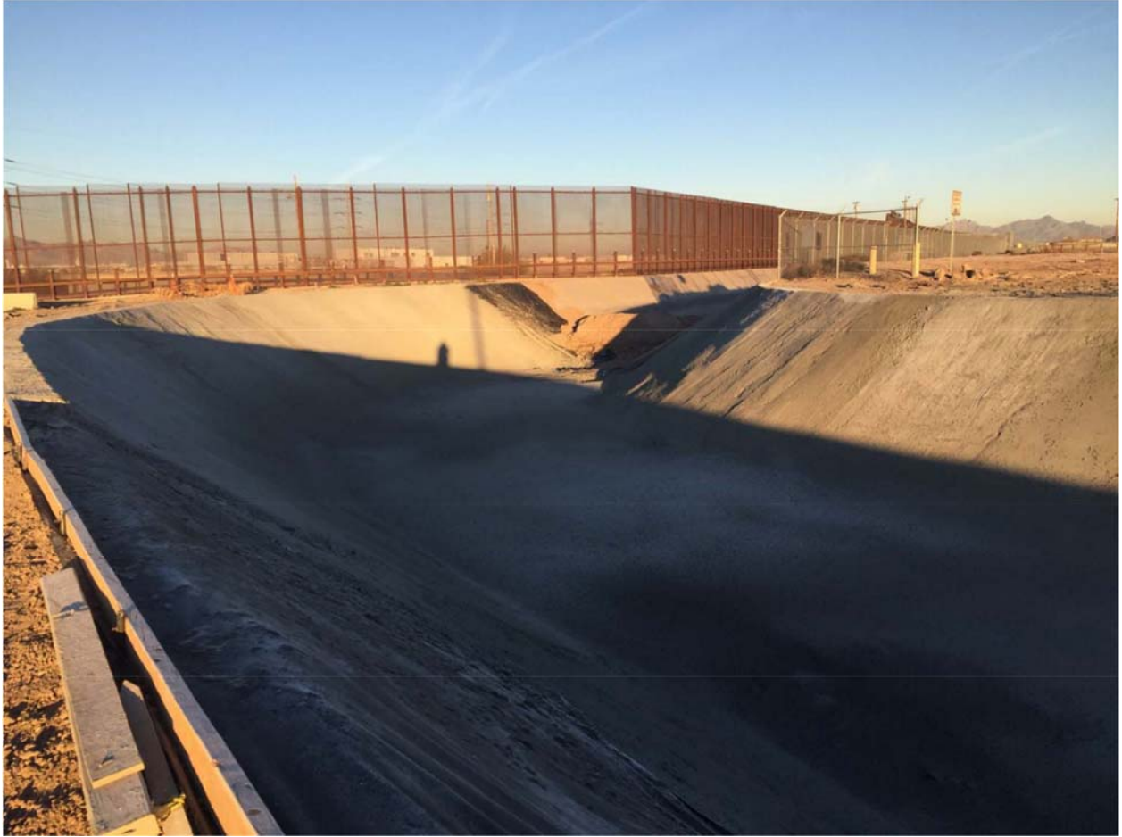
Location 1A. Canal sides and bottom were concrete lined. Photo dated 1/21/16.
