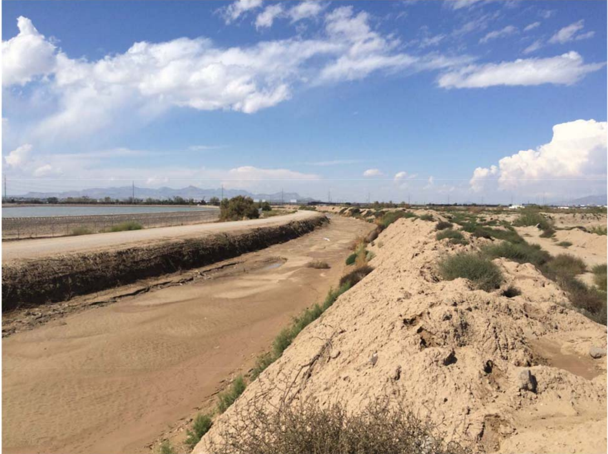
Location 5. Pre-construction photo dated 10/21/15 of the Riverside Canal approximately 2,000 feet from the heading. Piled dirt on the left bank was used to prevent overtopping.
