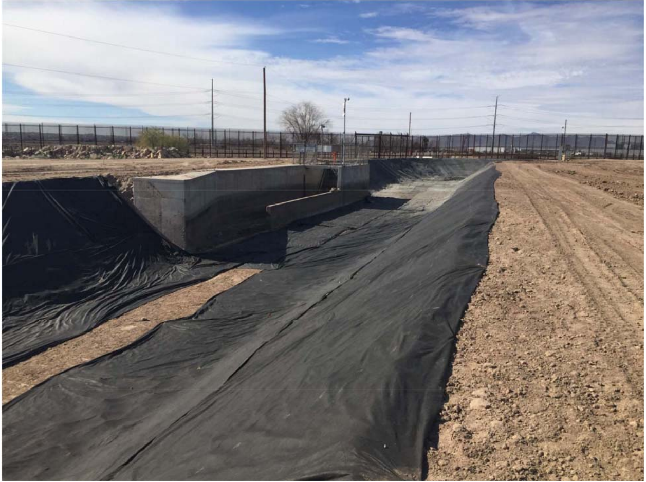
Location 2. Geofabric liner placed on both canal banks. Photo dated 1/15/16.
