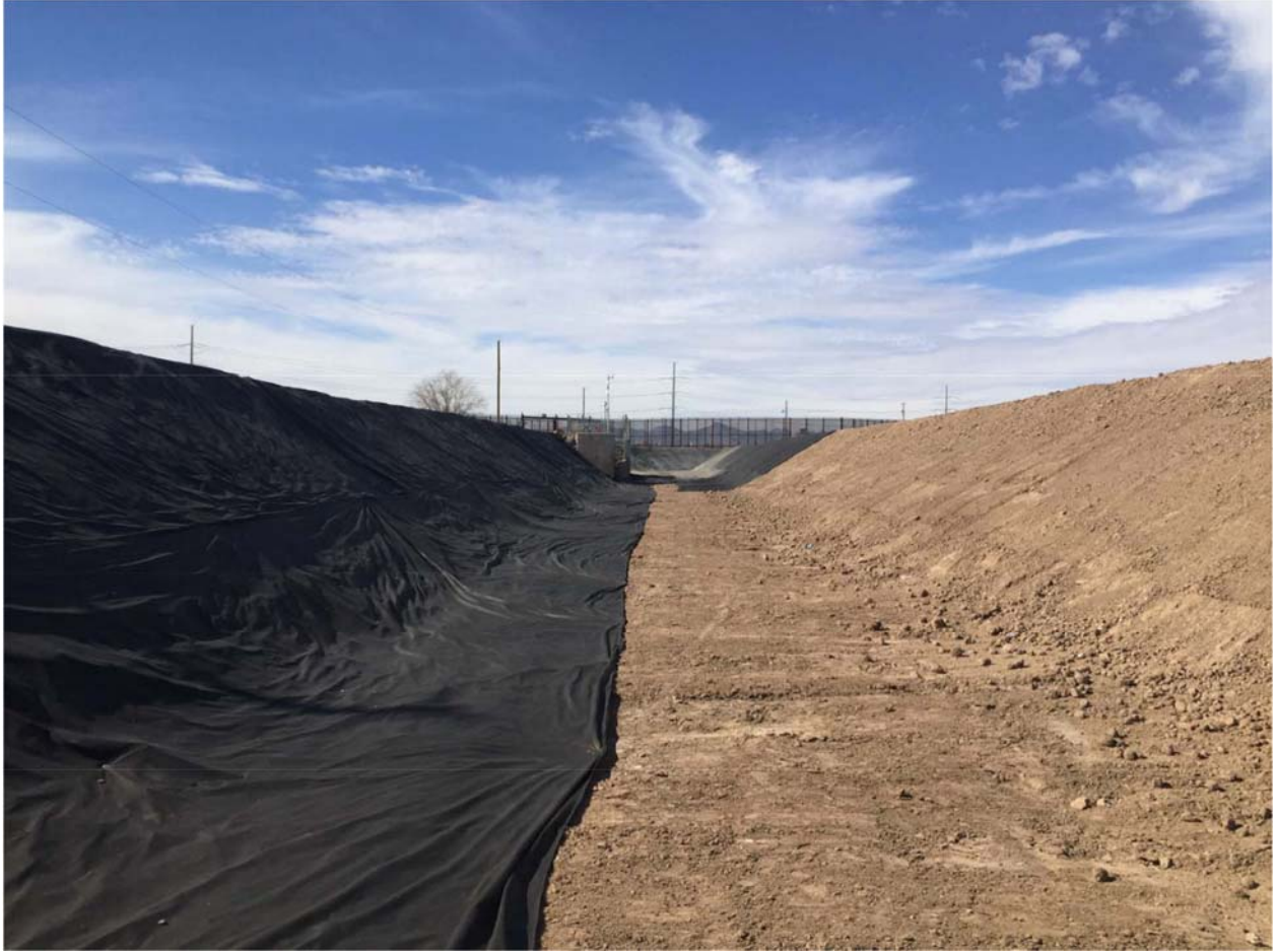
Location 3. Geofabric liner placed on the right canal bank. Photo dated 1/15/16.
