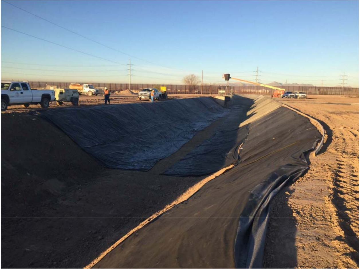
Location 4. Geofabric liner placed on canal sides. Photo dated 1/21/16.
