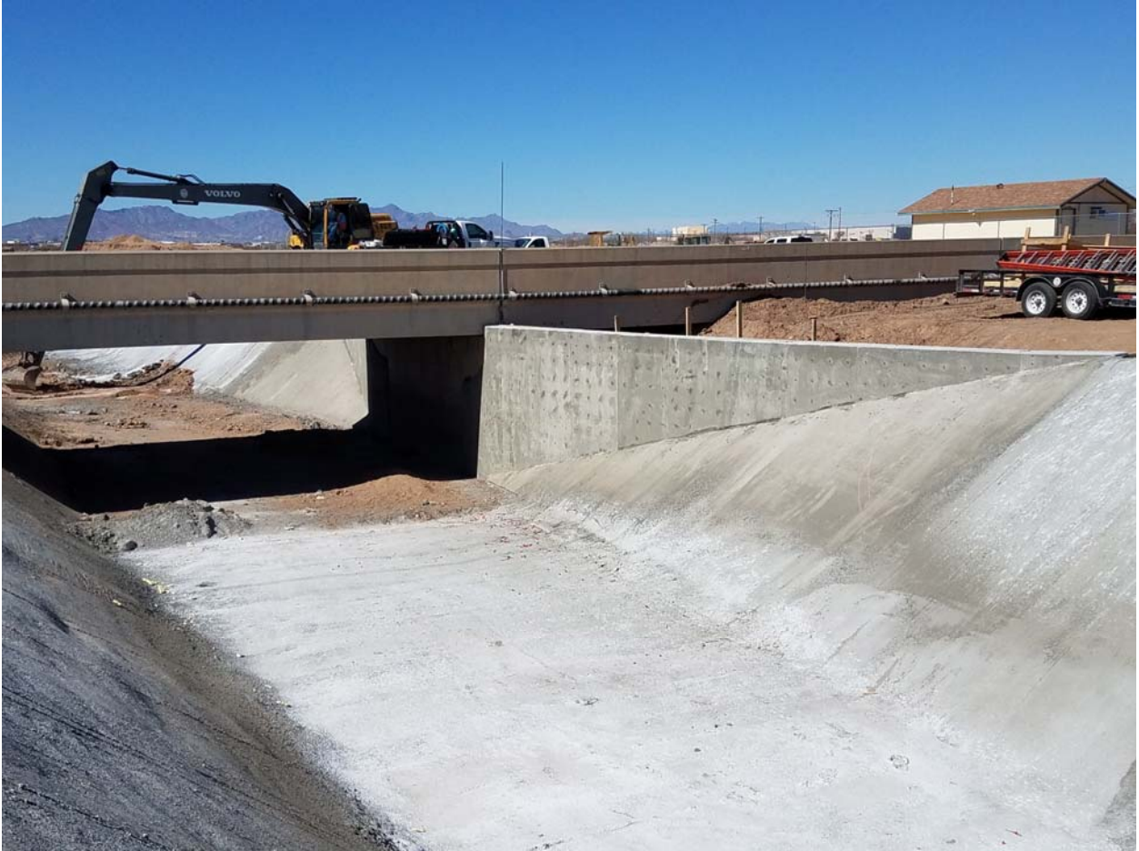
Concrete lining in progress downstream from the Pan-American Bridge. Photo dated 2/20/17.
