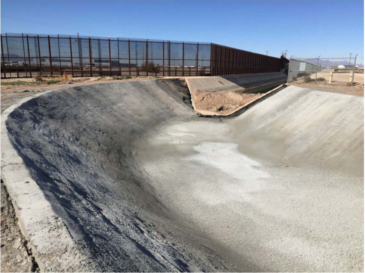
Location 1A. Dried shotcrete at Riverside Canal heading. Photo dated 2/4/16.
