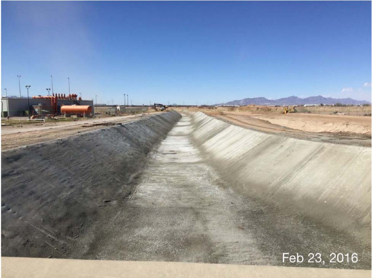
Location 6. Concrete lining was completed at this location. Photo dated 2/23/16.
