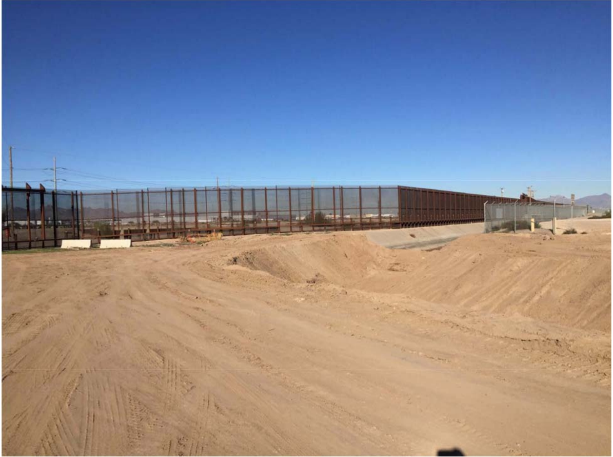
Location 1A. Earthwork and canal shaping completed. Photo dated 11/18/15.
