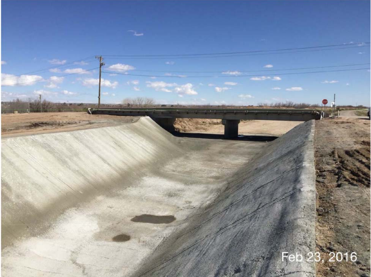
Concrete lining was completed at the Pan-American Bridge. Photo dated 2/23/16.
