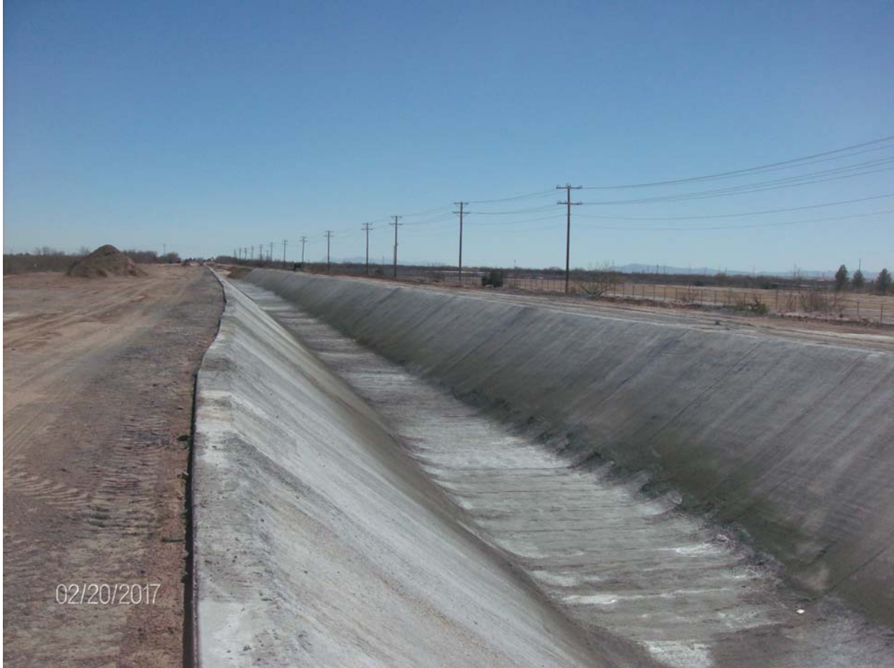
Concrete lining completed downstream from the Pan-American Bridge. Photo dated 2/20/17.
