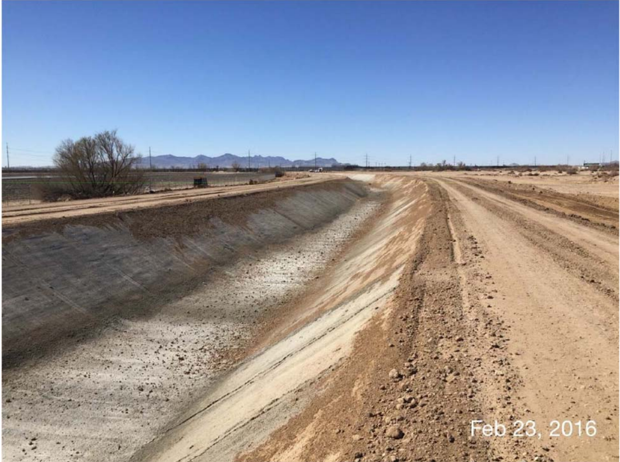
Location 5. Concrete lining was completed at this location. Photo dated 2/23/16.
