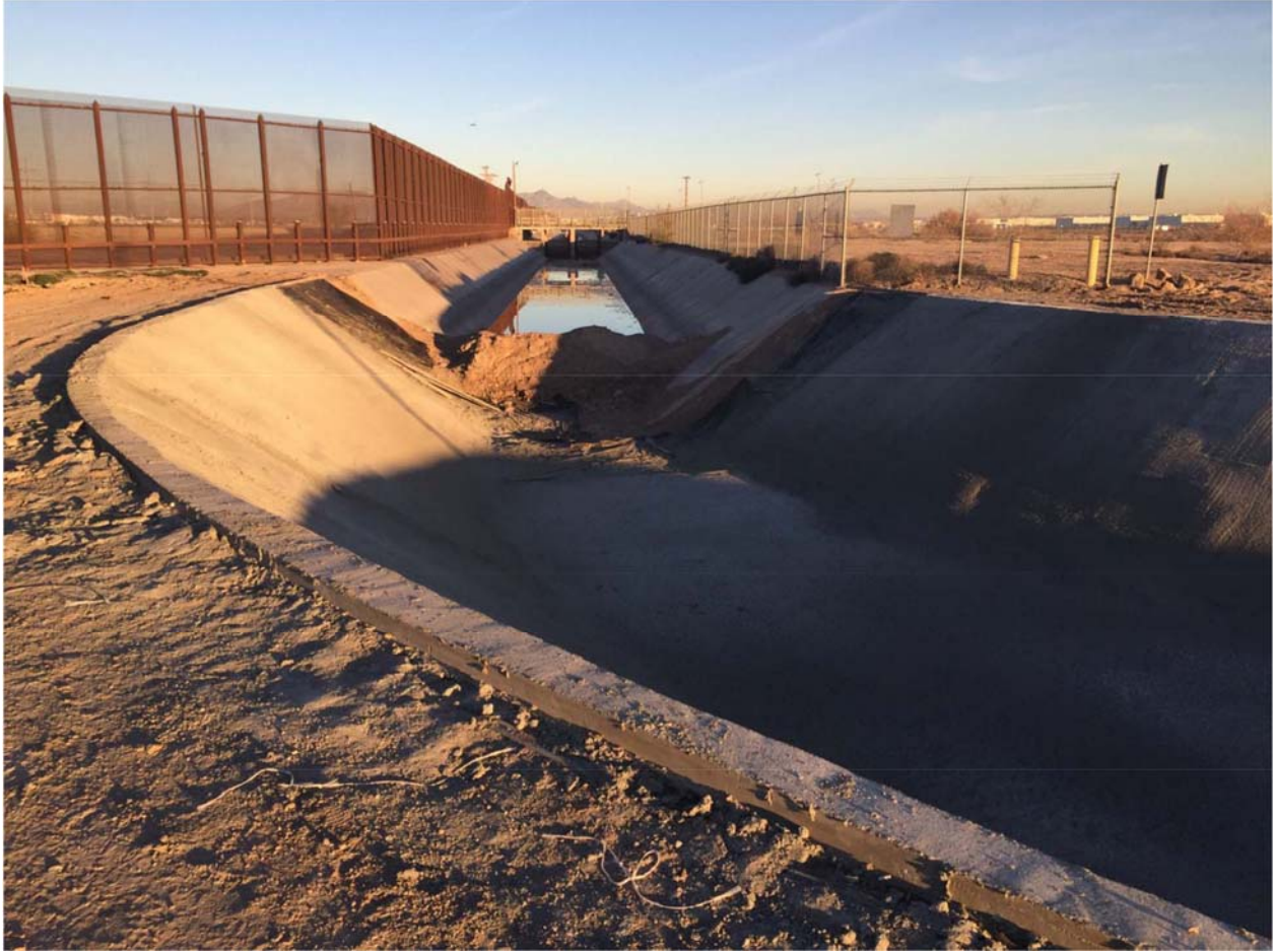
Location 1B. Canal sides and bottom were concrete lined. Photo dated 1/21/16.
