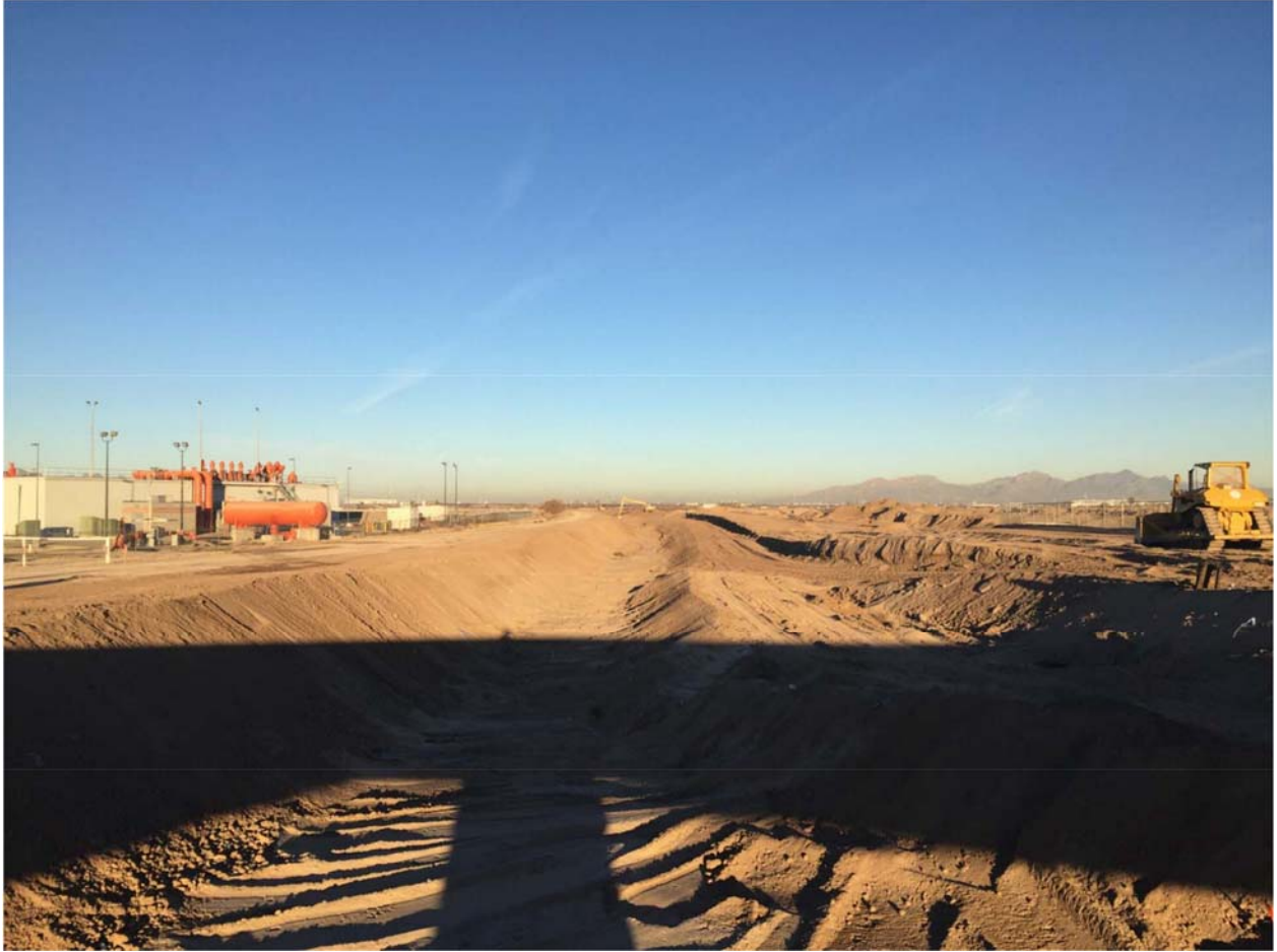
Location 6. Continued earthwork and canal shaping. Photo dated 1/21/16.
