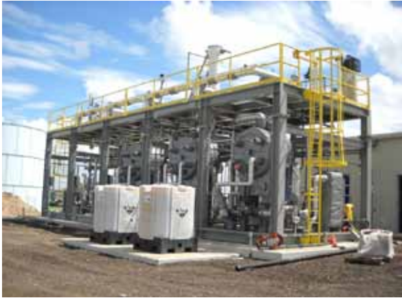
Figure 31. Laredo Site Assembly Complete
