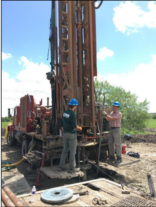
Figure 9. USGS staff logging the borehole to a total depth of 1,095 ft. Photo taken 8/19/2016.
