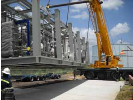
Figure 29. Skid Base Installation
