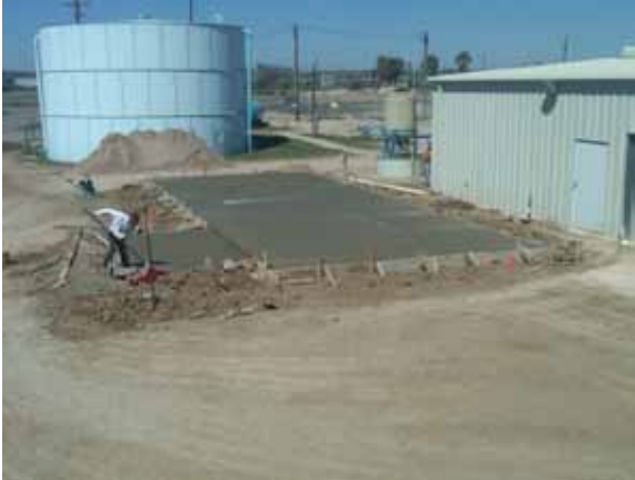
Figure 28. Completed AdVE Concrete Pad Adjacent to RO Plant Building
