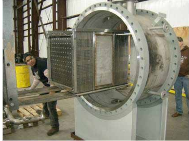
Installing Plate Pack
