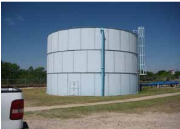
Figure 23. Finished Water Tank
