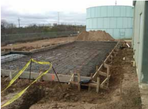
Figure 27. AdVE Skid Concrete Pad Framing
