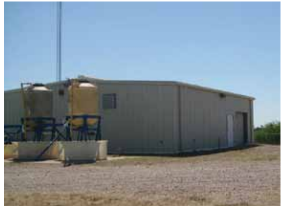
Figure 24. RO Plant Building
