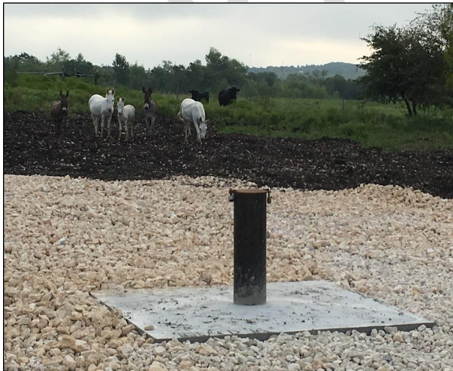
Photograph of completed Multiport well on 9/13/2016.
