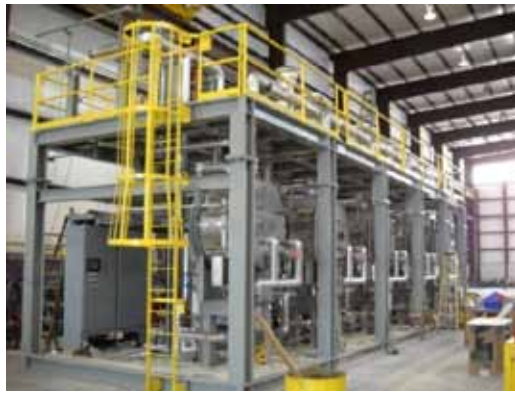
Figure 12. AdVE Laredo Pilot Plant at TSC Prior to Insulation
