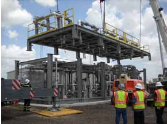
Figure 30. Skid Upper Platform Installation
