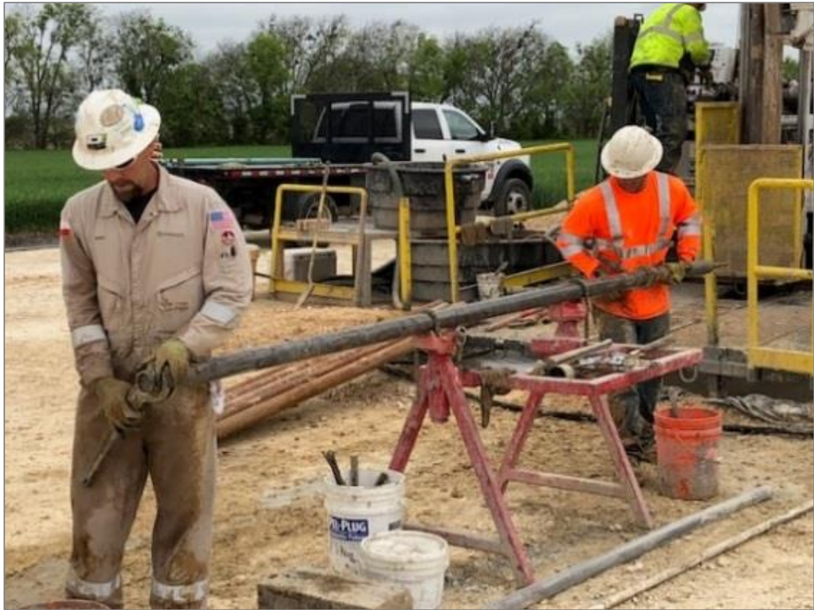
Figure 2-4: 2.5-inch core being removed from tool
