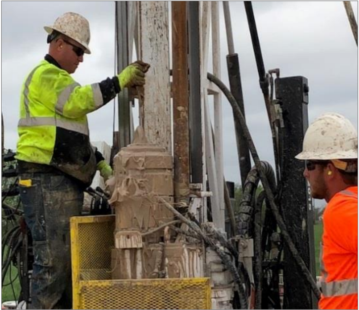
Figure 2-3: Closeup of coring operation
