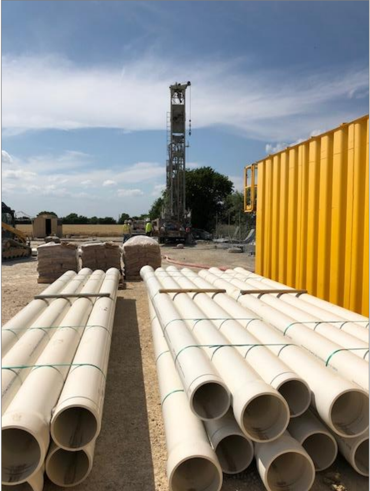
Figure 2-10: SDR 17 casing pipe
