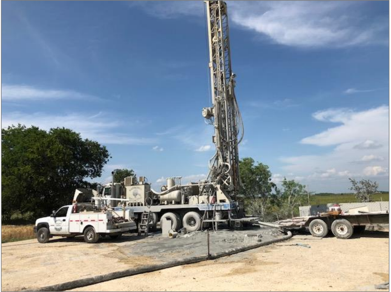
Figure 2-9: Kutscher drilling rig
