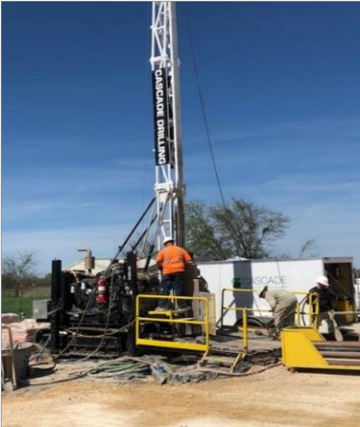
Figure 2-2: Cascade drilling rig
