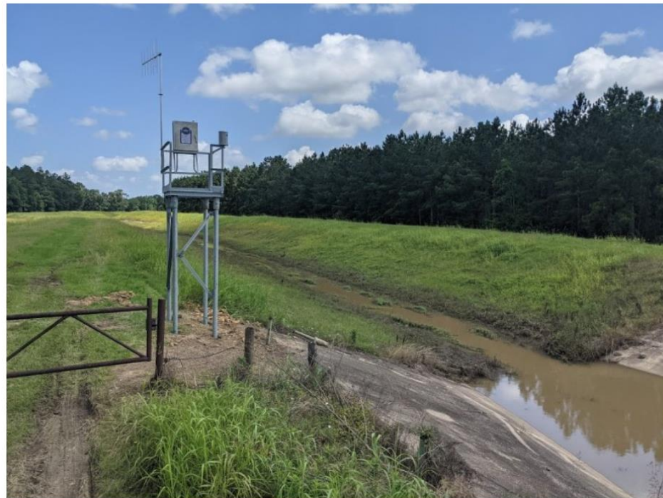
New elevated ALERT II station
