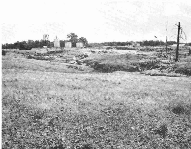
A. Oil well site showing brine pollution which is killing vegetation and contributing to soil erosion (East Texas oil field near site 15)
