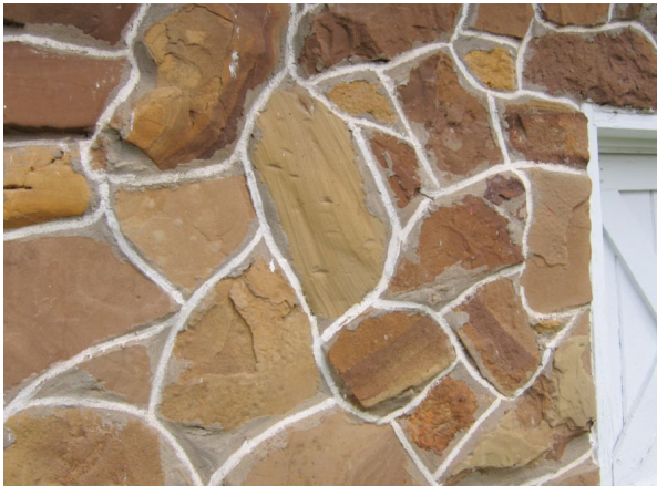
Part of the Rockdale Chamber of Commerce building built from sandstone of the Carrizo Formation.
