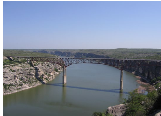
Looking north at the Pecos River Bridge and the Devils River Limestone along U.S. Highway 90.
