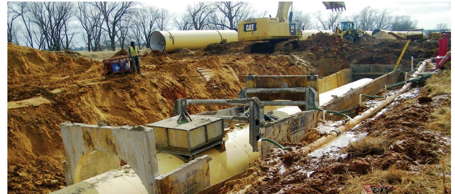
SWIFT-funded pipeline under construction.
